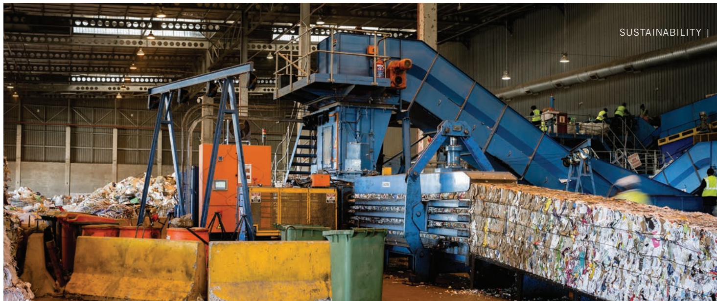
Recovered paper at a material recovery facility in Cape Town where the material is sorted, compacted and baled.
