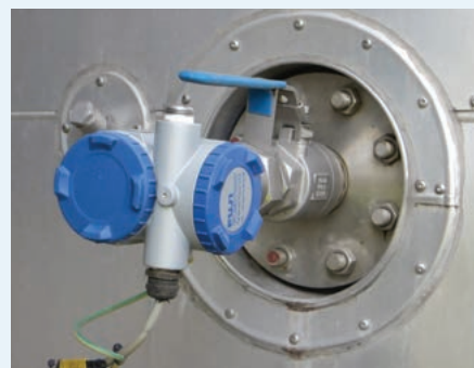
Fuji level and pressure transmitters with ball valve design at Cristal Union's manufacturing plant in Aulnat, central France. Maintenance teams don't have to take the tank out of service to remove the transmitter for maintenance.
