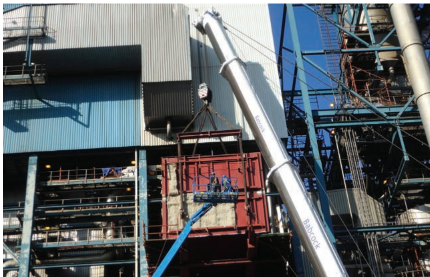
CLOCKWISE FROM TOP LEFT. 50t and 500t mobile cranes with 500t positioning the economiser boxes for welding; installation of new economiser banks, 3 and 4, using LTM1500 with guyed main boom of 42m; removal of old economiser banks 1 and 2, with a weight of 116t using LTM1500 with guyed main boom.
