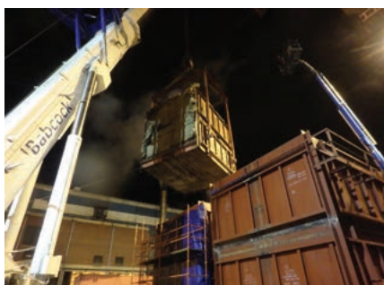
CLOCKWISE FROM TOP LEFT. 50t and 500t mobile cranes with 500t positioning the economiser boxes for welding; installation of new economiser banks, 3 and 4, using LTM1500 with guyed main boom of 42m; removal of old economiser banks 1 and 2, with a weight of 116t using LTM1500 with guyed main boom.
