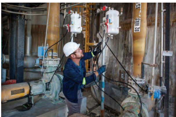
Continuous loop flushing and lubricating systems supplied by AESSEAL, fitted to pumps at Mondri Richards Bay.
