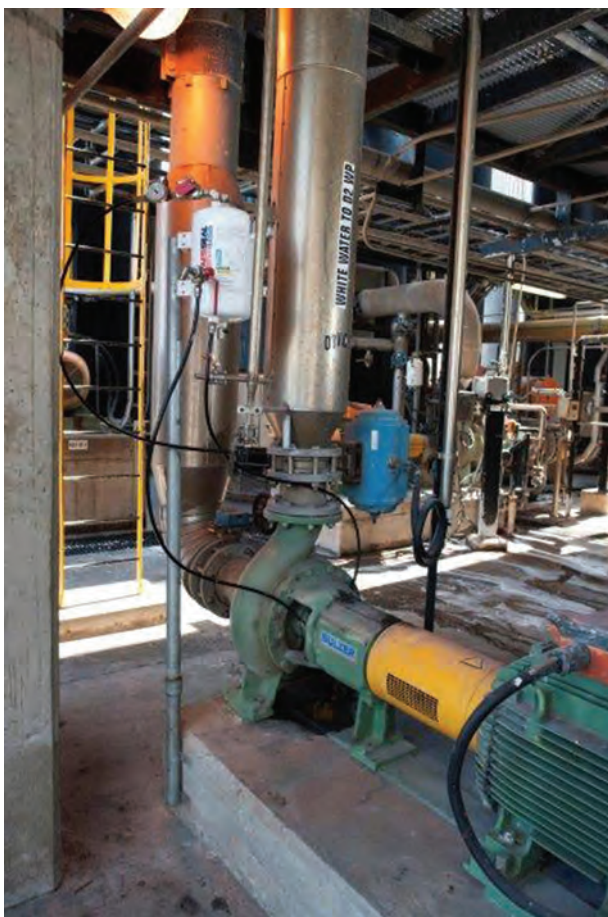
After: Pump and mechanical seal at Mondri Richards Bay, fitted with AESSEAL continuous loop flushing and lubricating system.
