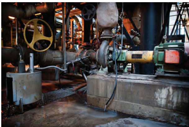
Before: Pump and mechanical seal at Mondri Richards Bay, fitted with quench-to-drain flushing system.
